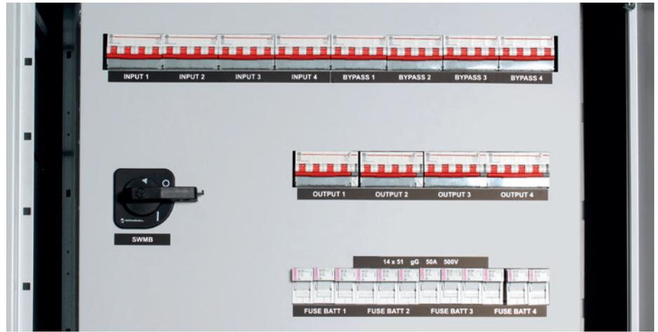
Detail of protective devices and disconnectors
