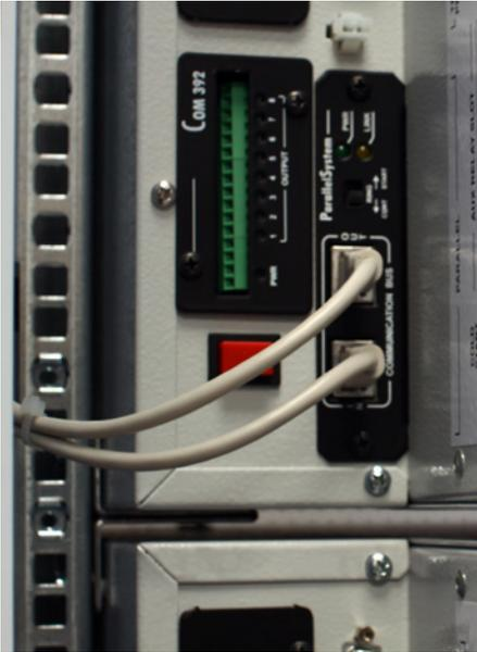
Parallel configuration and programmable relay contacts board
