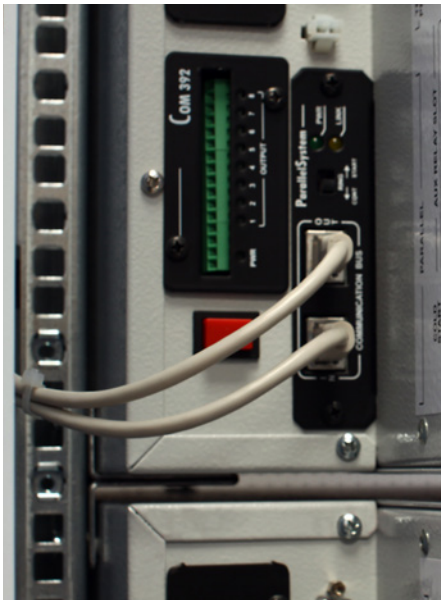
Parallel configuration and programmable relay contacts board
